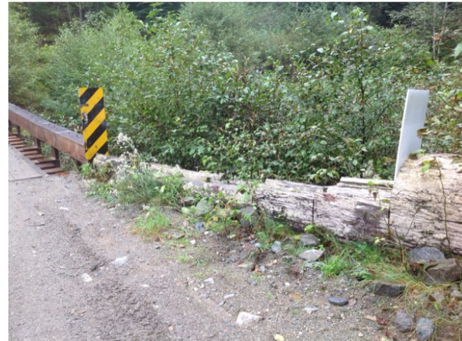
upstream left approach fender
