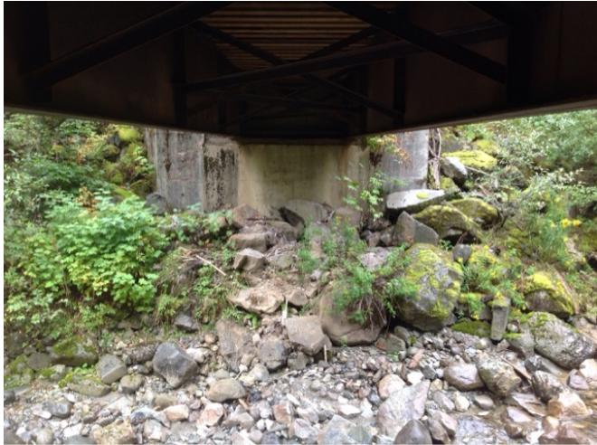
Right Bank Abutment when facing downstream
